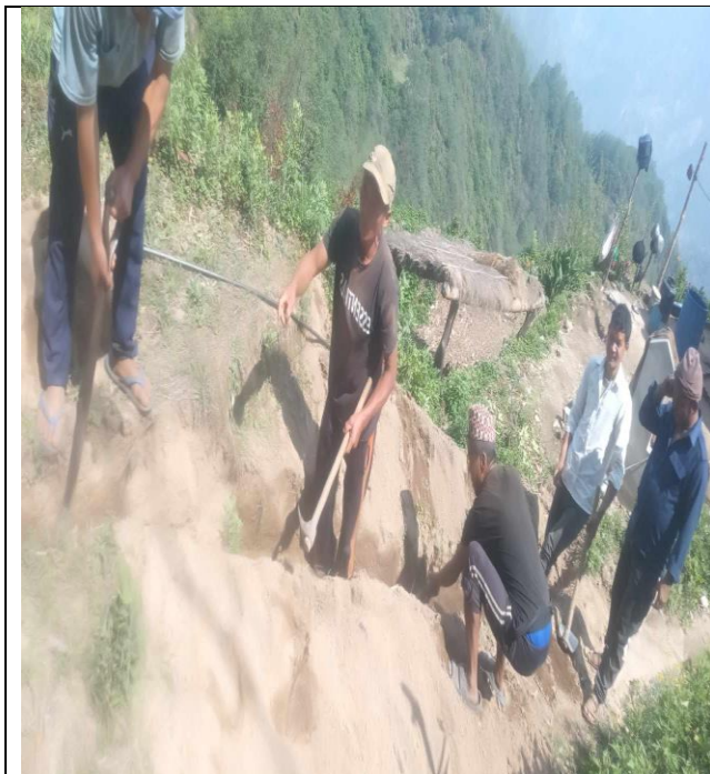
Pipe line- 5300m
